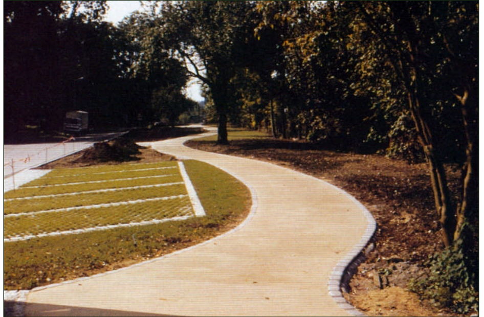
Lanes, close to nature, prenable to water and air made of Durocs 1120 and sand.
