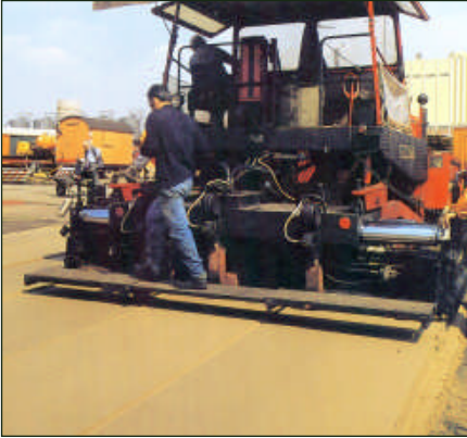
Lanes, close to nature, prenable to water and air made of Durocs 1120 and sand.
