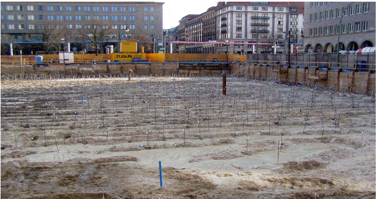
Bottom sealing with PURSEAL 912
